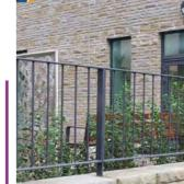
Steel Balustrade - Protective barrier where fall is > 600mm
